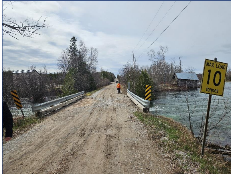
Photograph 17: Looking south across the structure.
