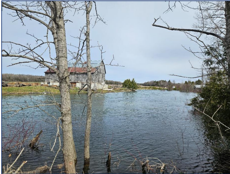
Photograph 1: Looking north upstream of the bridge site. Water backwater is pushing up into the trees along the roadway.
